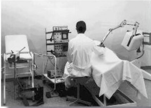
An early articulated-arm compound static scanner from Kretz Technik, Austria** A vaginal scanning device is seen on the left
